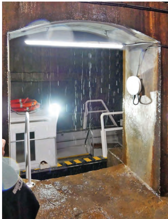
Emergency access adit, showing modern reinforcements. Photo Gerald Tompsett
